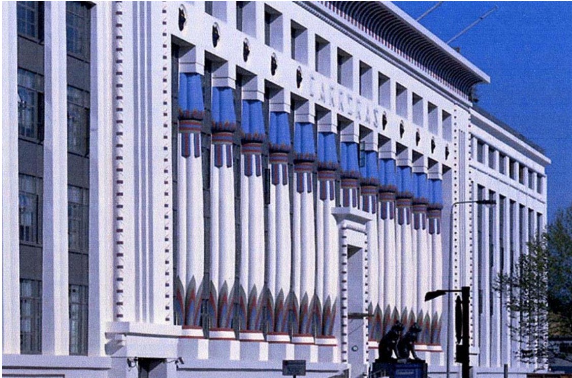
The restored Carreras factory with its guardian cats.
