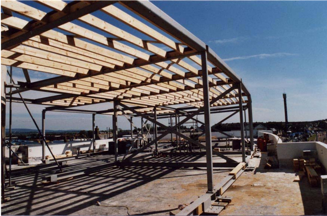
On the hotel roof the framework for the additional floor is nearing completion.
