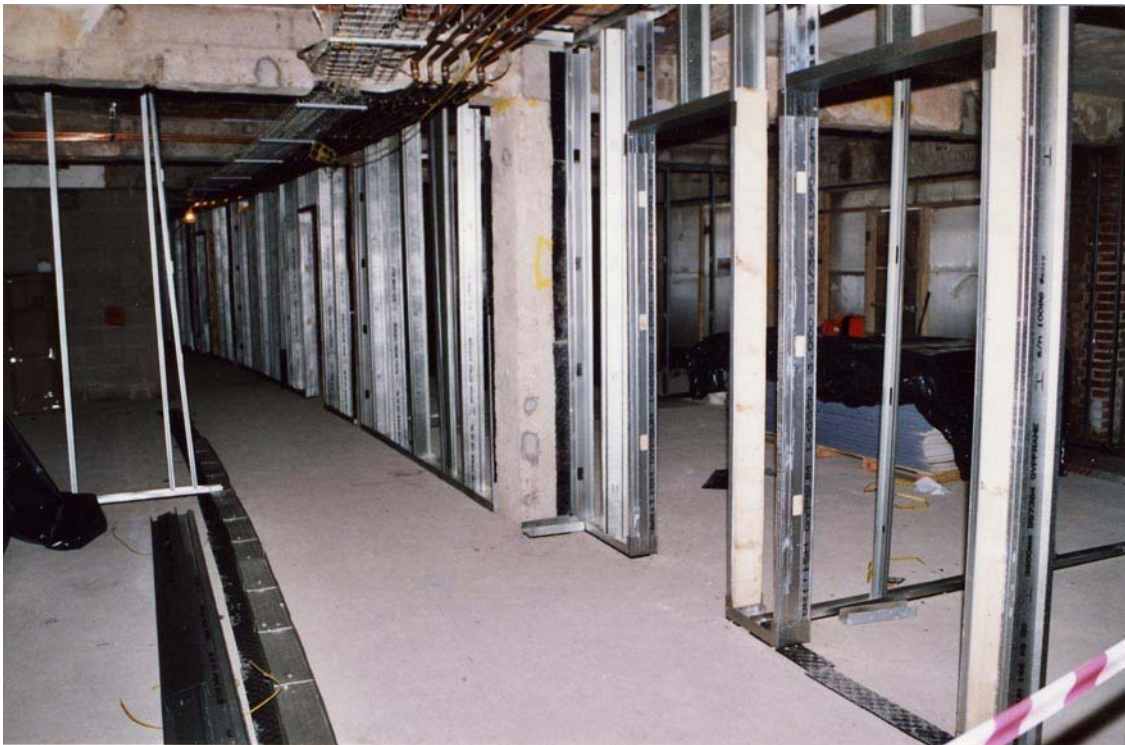
Inside, on the first floor, most of the partition walls for the bedrooms have been installed and plastering has begun.
