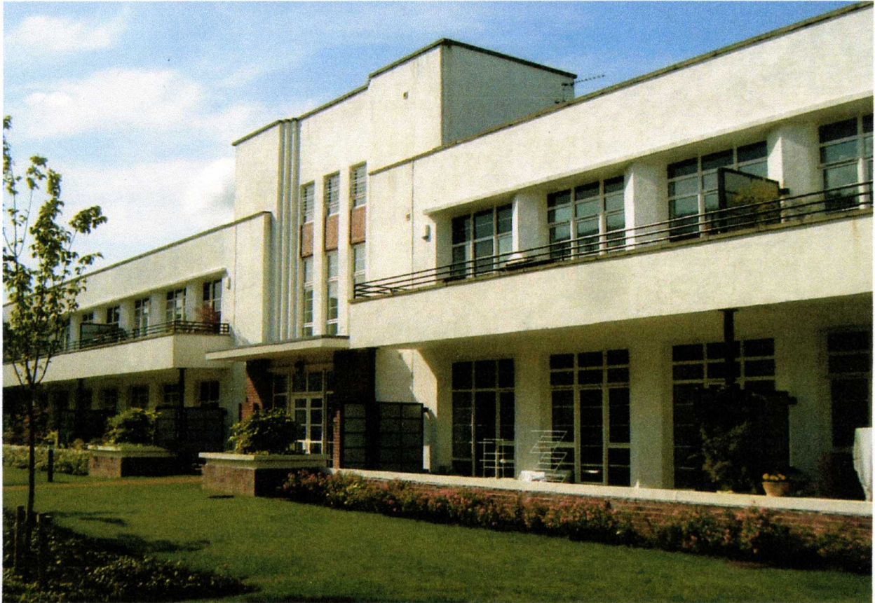
Canniesburn Hospital has been converted into apartments within a modern housing estate
